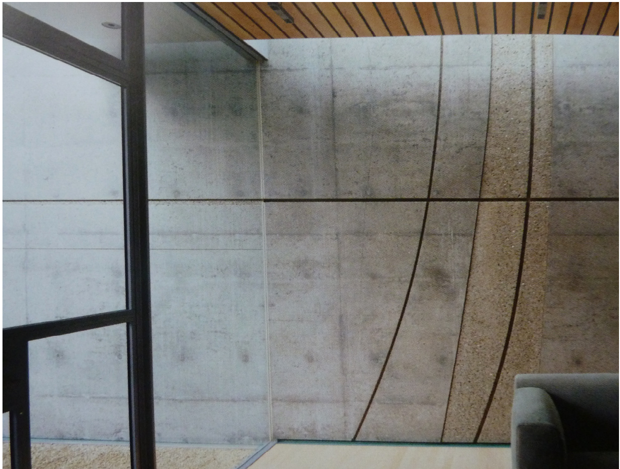
Mechanical intervention of a cast surface. The curved grid lines were cut into the surface and the exposed aggregates grit blasted. Visiting Artists House, California. Jim Jennings Architecture.
