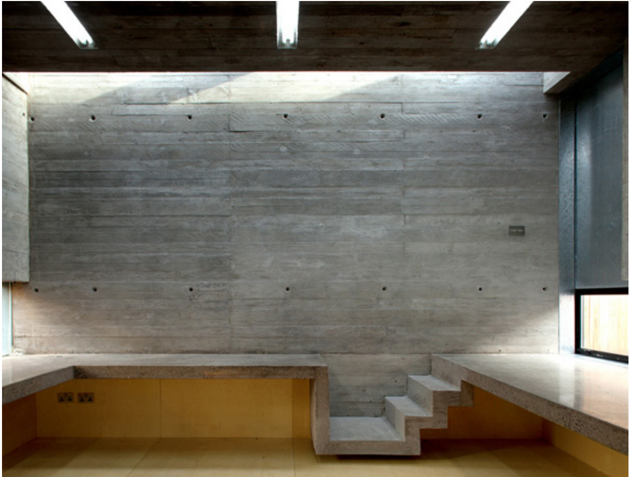
Board Marked Finish. With in situ polished and ground Flatwork. By Architecture Republic. Photo by Paul Tierney
