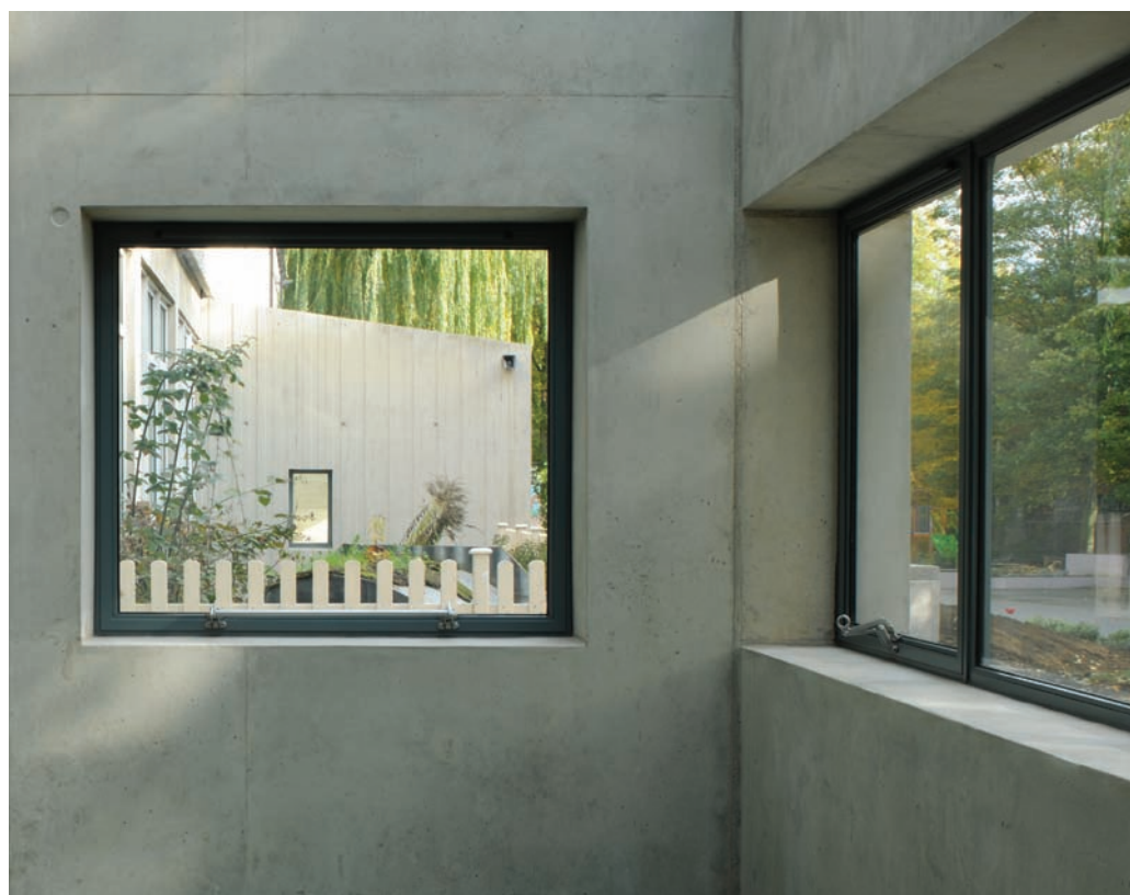
Above: Steel Crittall windows fill the exposed reveals.
